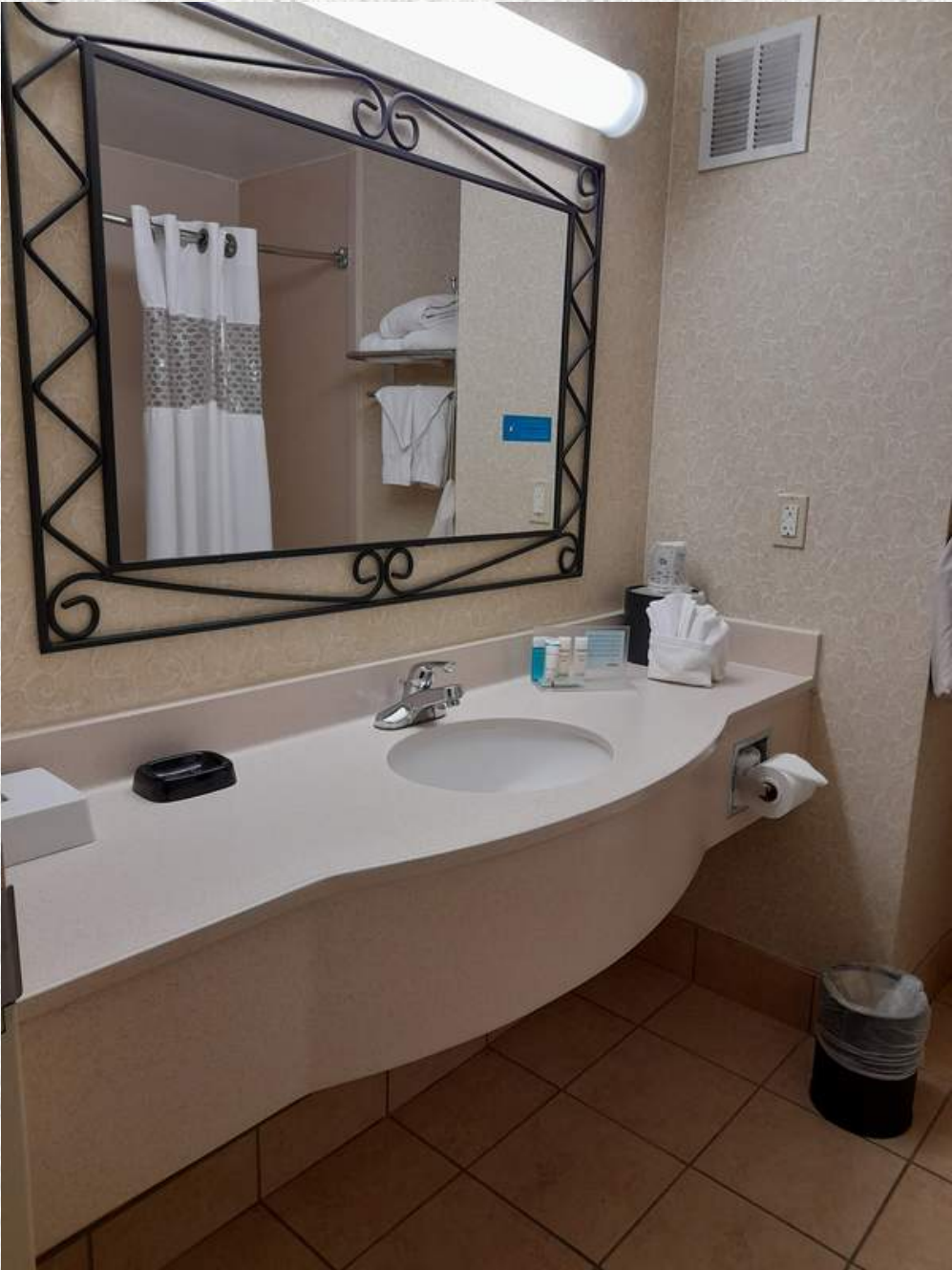
Another elegant, unique and custom hotel vanity installation.
